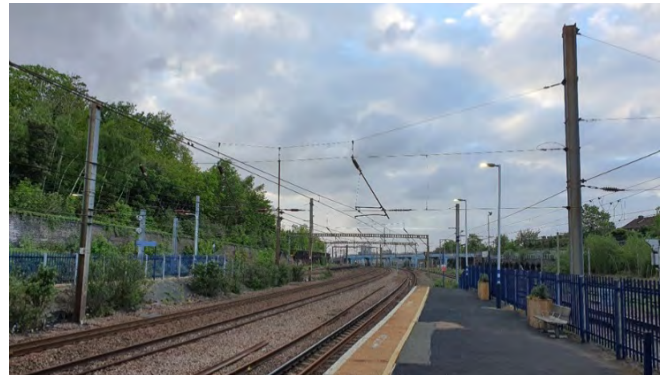
Figure 5: Portal OLE (left) and head span OLE (right) configurations
